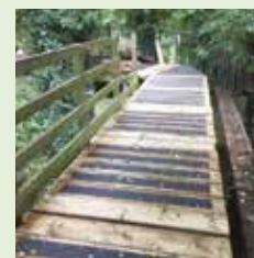
Part of handrail fixed
