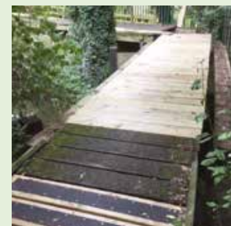
Walkway at far end to be completed
