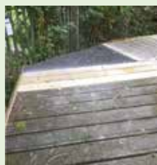
The grid in place
