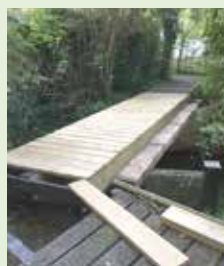
Boards placed on bridge
