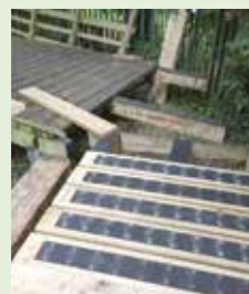
Non-slip panels added
