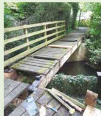
Hand rail removed
