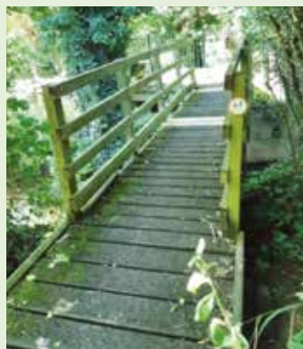
Bridge before works
